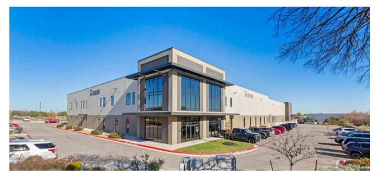
KDW completed construction of High Tech Flooring and Design's new headquarters in Austin, TX a 74,399 SF facility featuring a concrete tilt wall facade, structural steel core, and TPO roof. The 38,000 SF office space across two floors fosters collaboration and efficiency, while a prominent 7,500 SF showroom showcases High Tech Flooring's craftsmanship and products.
